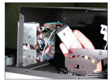
8 Pull the ballast out of the housing. Do not disconnect any wires at this time. The wires have enough slack to pull the ballast completely out without disconnecting.
