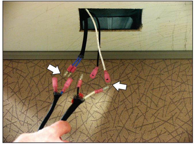
**9** Pull the transformer wires out until the terminals are accessible.
